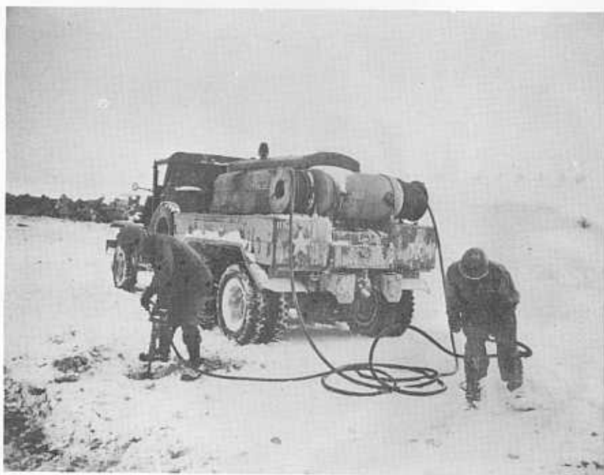
Men of 63rd Combat Engineers Battalion, 44th Infantry Division, prepare to blast holes in the ground, which is frozen to a depth of 18 inches, for artillery emplacements. Preparations are being made for emergency use of emplacements by 105 mm howitzers in Pauling area, France. 25 January 1945.
