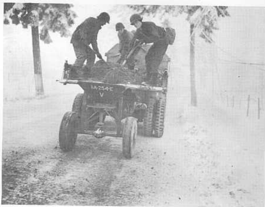
Men of 245th Combat Engineers use a sanding device made from a salvaged German vehicle on an icy road near Sourbrodt, Belgium, 7 January 1945.
