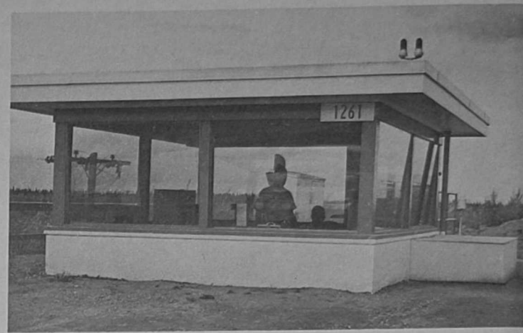
THE REPRESENTATIVE OBSERVATION SITE gives the observer an unrestricted view of the Eielson AFB flying facility.
