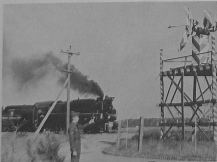
WIND VELOCITY reading from a portable wind set is taken by A2c Robert E. Shannon, at the crossroad of Felker Army Airfield's Ground Control Approach and the track of the Ft. Eustis Military Railroad.
