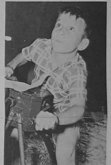
FUTURE weather observer operates the ML-121, portable ceiling light and generator, at the weather station at Ft Eustis, Va.
