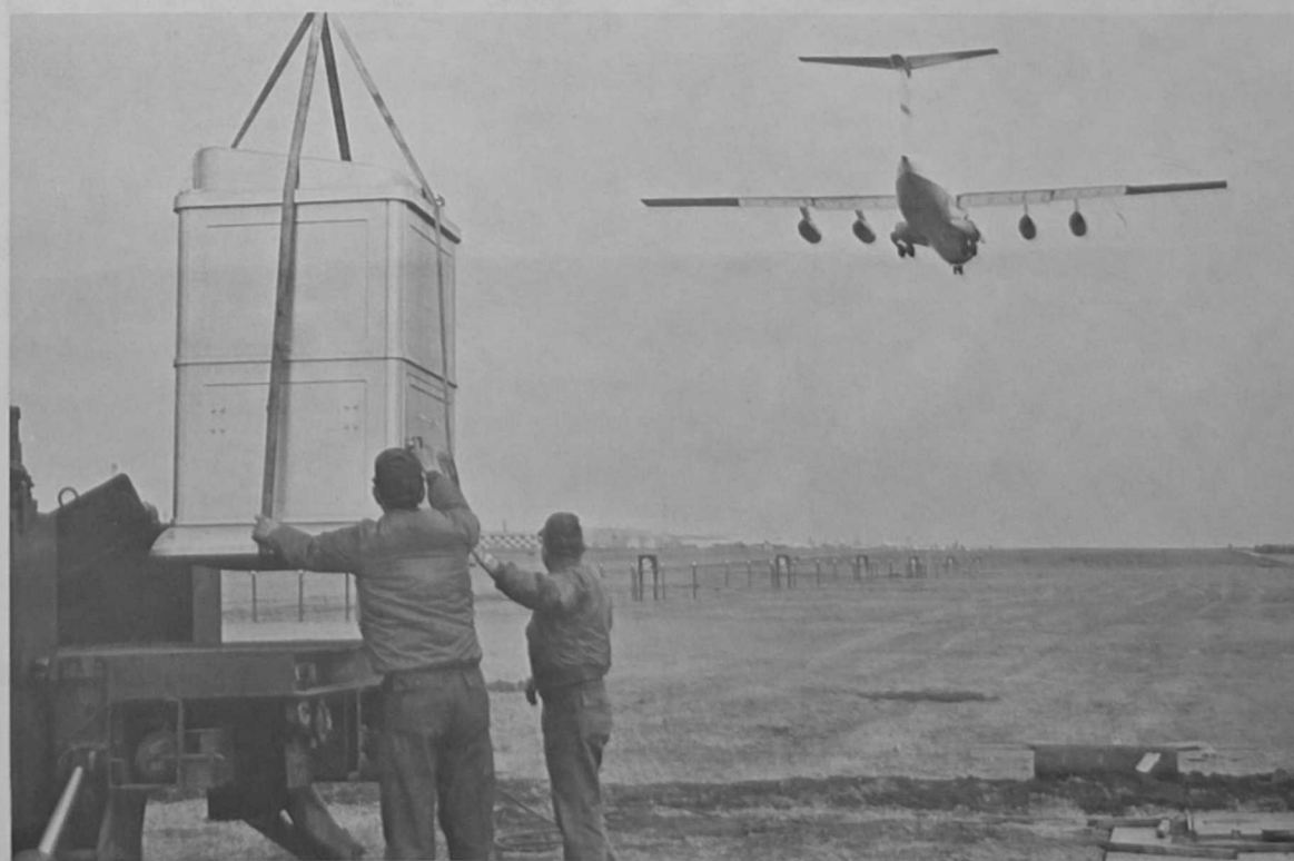
BULLS-EYE-- An illusion of pinpoint accuracy by a MAC combat airlift crew is created as the detector portion of an AN/GMQ-10 ceilometer is unloaded from a truck near the runway at Yokota AB, Japan. The relocation, attended by SSgt. David I. Diehl, left, and TSgt. James A. Burkhalter of the 1837th Electronics Installation Squadron, Air Force Communications Service, was made to improve the ceilometer's ability to measure very low clouds. (U.S. Air Force Photo by MSgt. Elliot D. Park)
