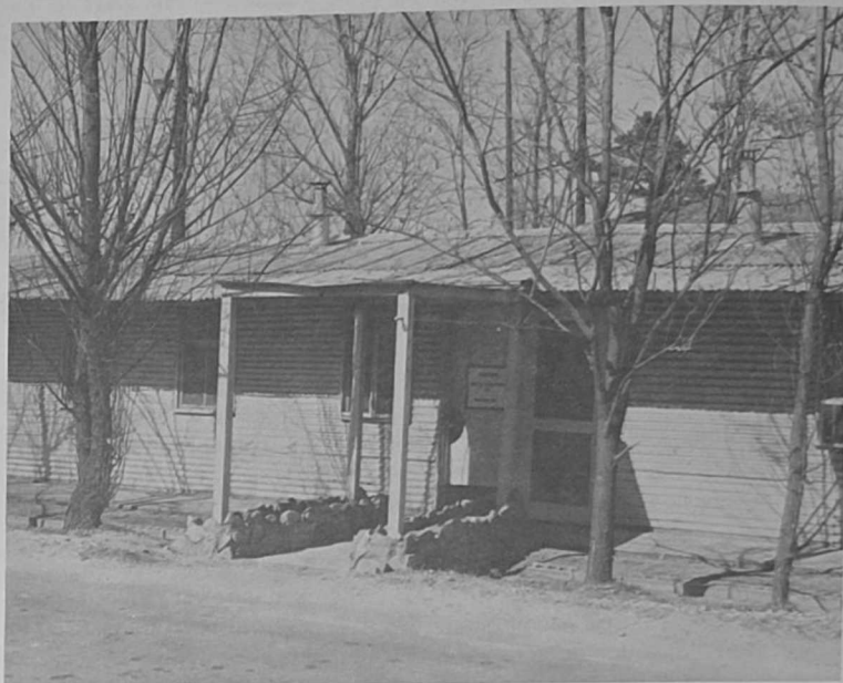
Outside view of building
