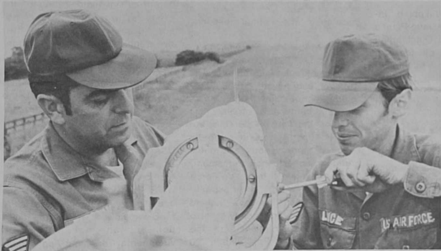
VISIBILITY INSTRUMENT - Technical Sergeant Andrew J. Fedornak (left) and Staff Sergeant Harold K. Luce repair a visibility measuring device - often used during the foggy English winters. The five-man maintenance section is responsible for the upkeep of $250,000 worth of equipment, including a tactical weather equipment kit which may be deployed with a forecaster and observer to any location where weather support is not available but is needed to support tactical operations. (U.S. Air Force Photo)
