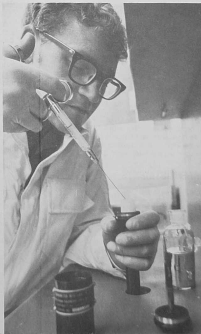
THE DELICATE TOUCH is what SSgt. Rick Hovarter gives an RVR-400 computer power supply he repairs.
