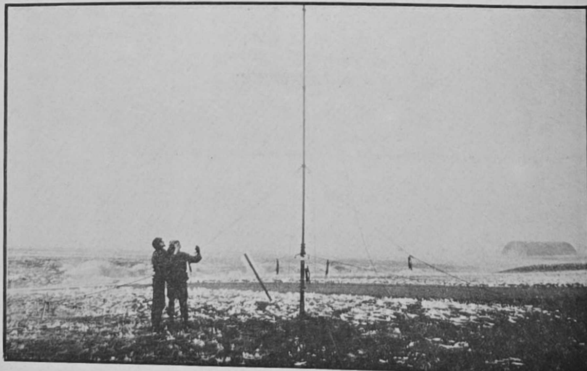
Amn. Michael Pickerign and SSgt. K.G. Smith put on the finishing touches and raise the GOLDWING antenna. The GOLDWING system receives worldwide high frequency weather data broadcasts.
