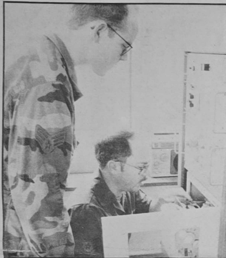
TSgt. John Hunrath, right, of the 1849th Engineering Installation Squadron, McClellan AFB, Calif., shows Sgt. Robert Manes of Det. 26, 7th Weather Squadron at Wiesbaden, the internal components of a newly installed wind recorder unit. The wind recorder was just one of the new instruments installed in the squadron recently. (U.S. Air Force photo by Sharon Gordon)
