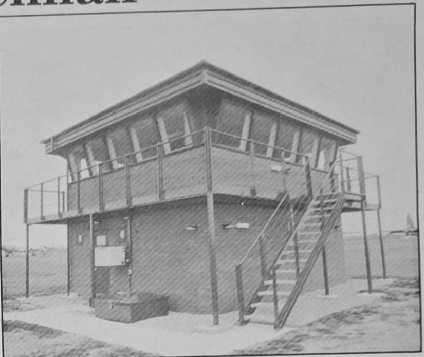
New ROS RAF Mildenhall, United Kingdom—view from the runway side.
