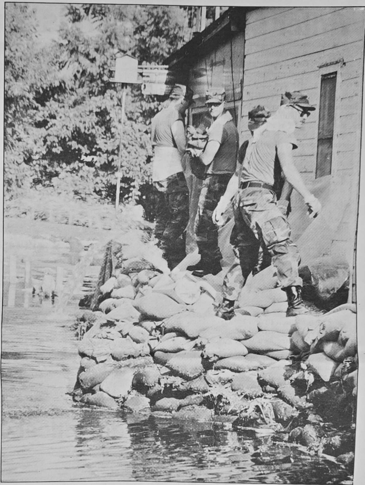
A group of Air Weather Service personnel rebuild a sand bag wall.
