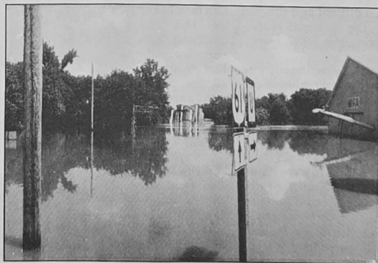
The bridge in the background was the only way to the community of Kaskaskia Island, Ill. For weeks barges and boats were the only transportation available.
